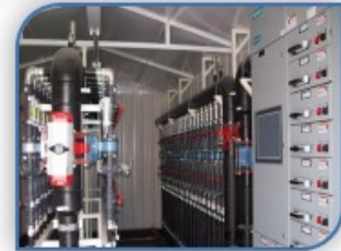
Interior of Header House
