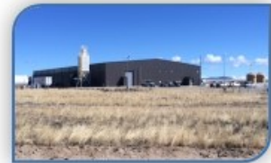
Lost Creek Plant
