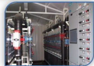
Interior of Header House
