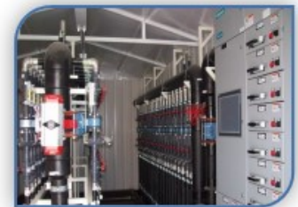
Interior of Header House
