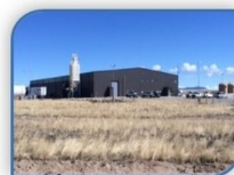
Lost Creek Plant
