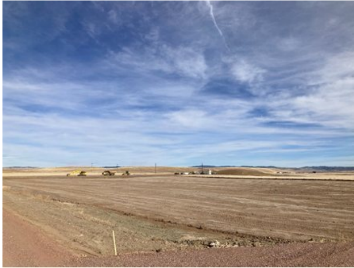
Initial topsoil stripping and compaction for the Shirley Basin satellite plant.
